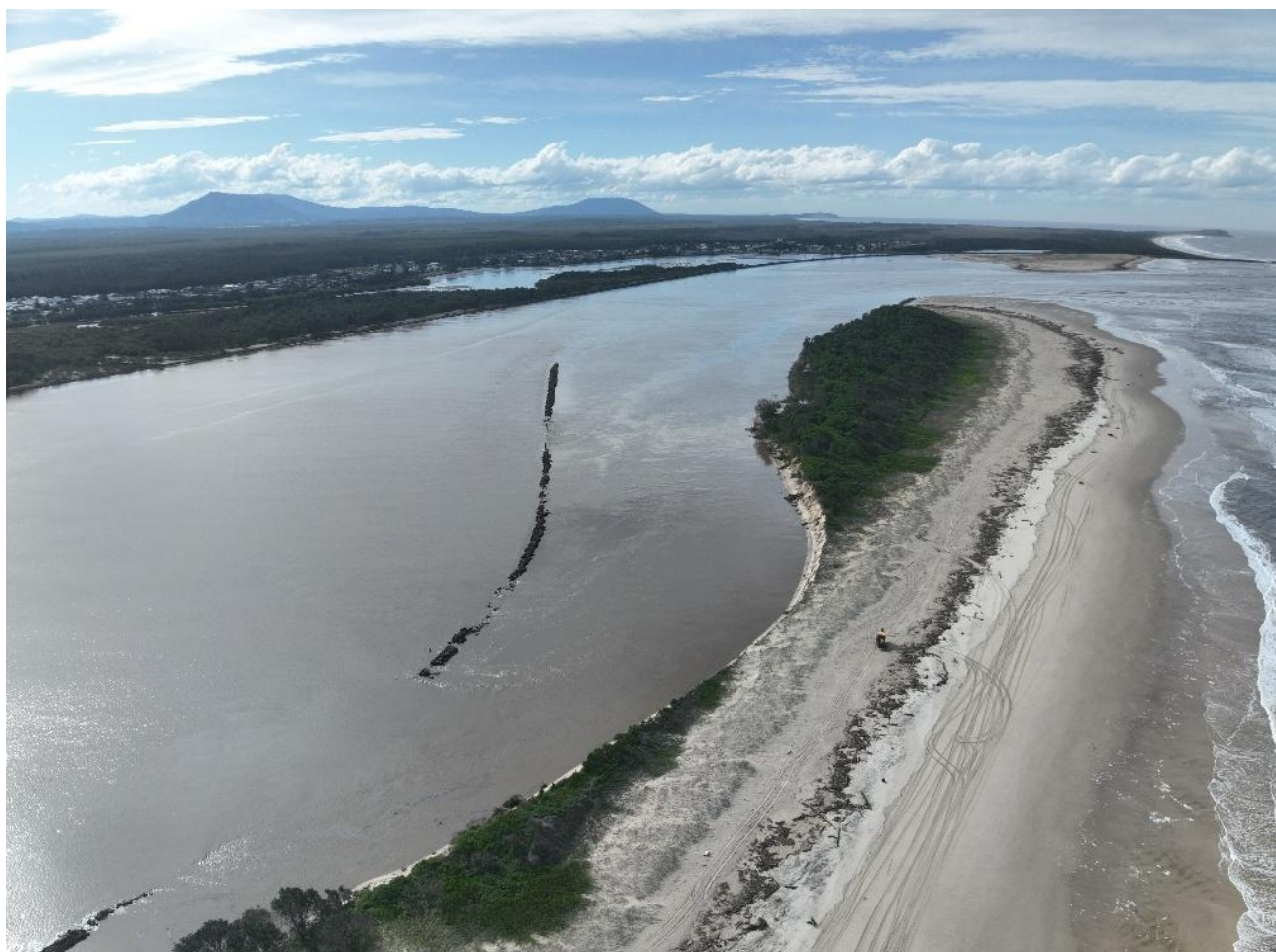
Figure 4: Damaged spur wall and breakthrough risk location.
