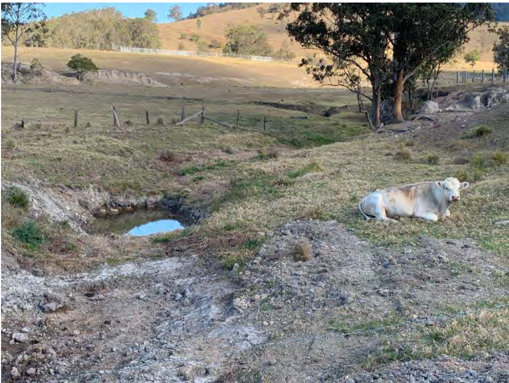
Photo 63 Avon River catchment – unnamed creek, site 123-03. Cattle access and minimal riparian vegetation. Gully erosion and bare eroding hills.
