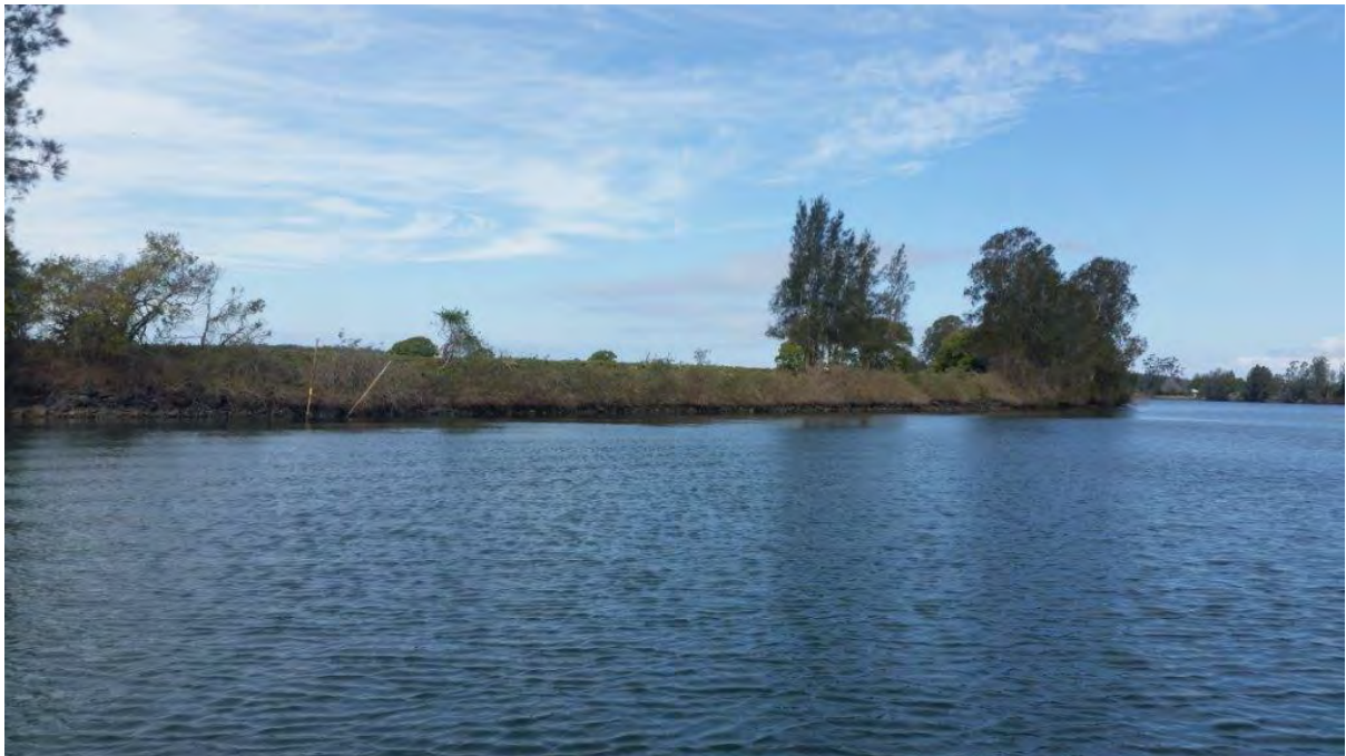
Photo 116 Manning River South Channel (Oxley Is. subcatchment 210). Pastures, no fencing. Steep banks with minimal riparian vegetation, exotic shrubs. Eroding banks.
