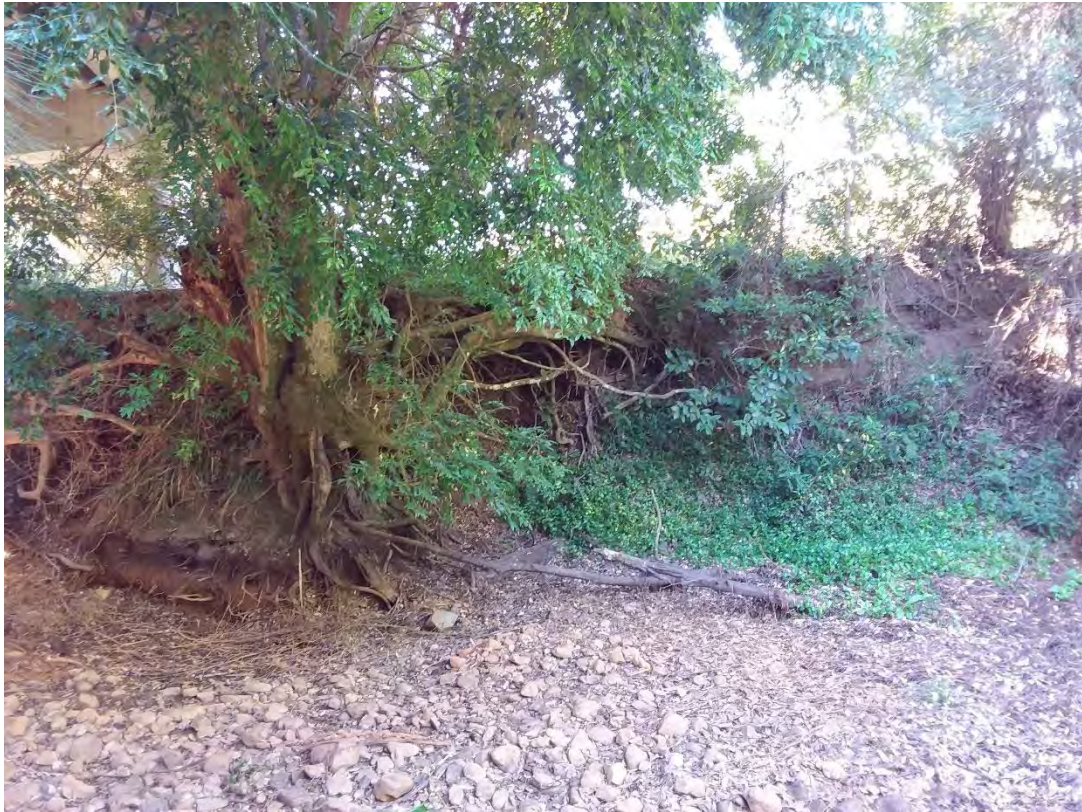
Photo 68 Burrell Creek - Bo Bo Creek Buckets Way crossing, site 113-05. Eroding vertical banks and exotic shrub and ground cover vegetation.
