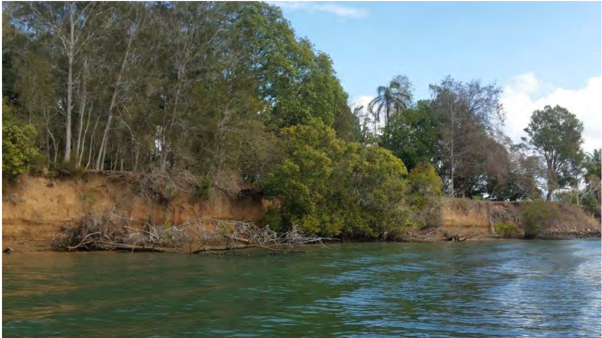
Photo 113 Manning River South Channel (subcatchment 114). Heavy erosion of banks has led to loss of riparian vegetation (Photo 111)
