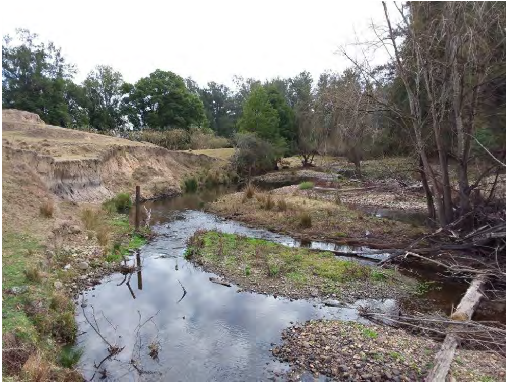
Photo 56 Gloucester River – near Gloucester Sewage Treatment Plant, site 122-03
